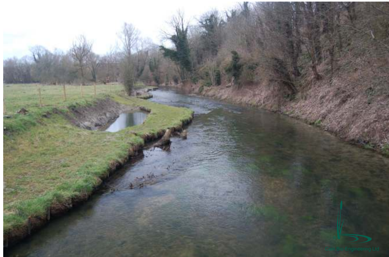
Sinuous flood berm with bio-diverse riparian zone
