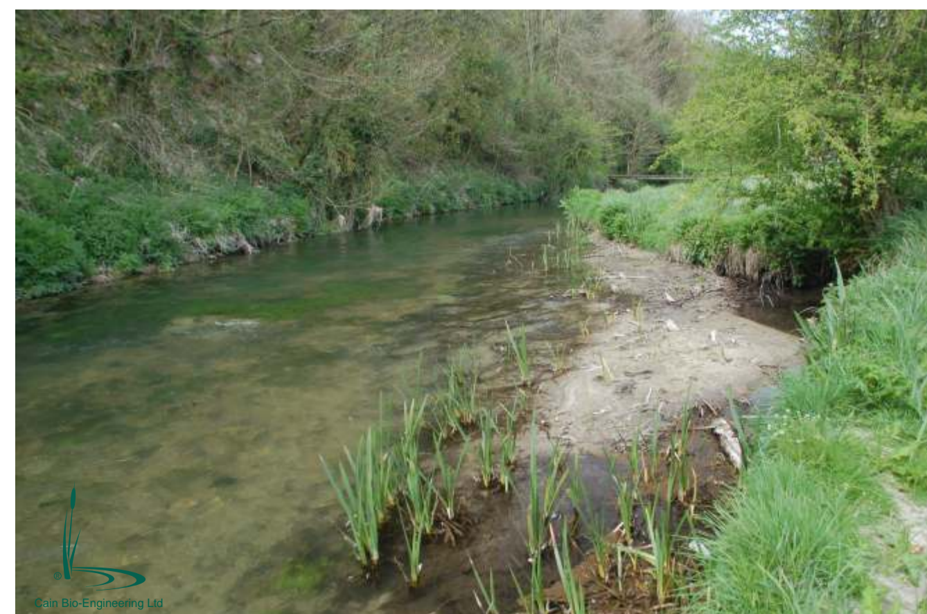
Brushwood sediment trap
