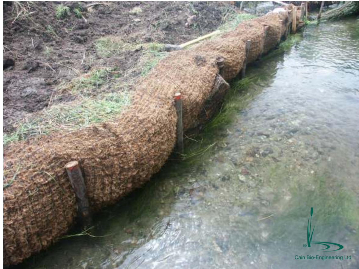
Coirnet bank revetment
