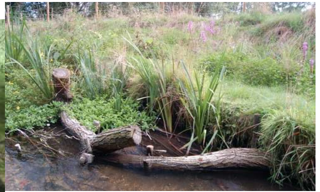
Fig.7a (above) The same structure 12 months later. This illustrates the way in which protruding sections of LWD & CWD can be combined with coirnet access banks to create sustainable marginal habitats.
