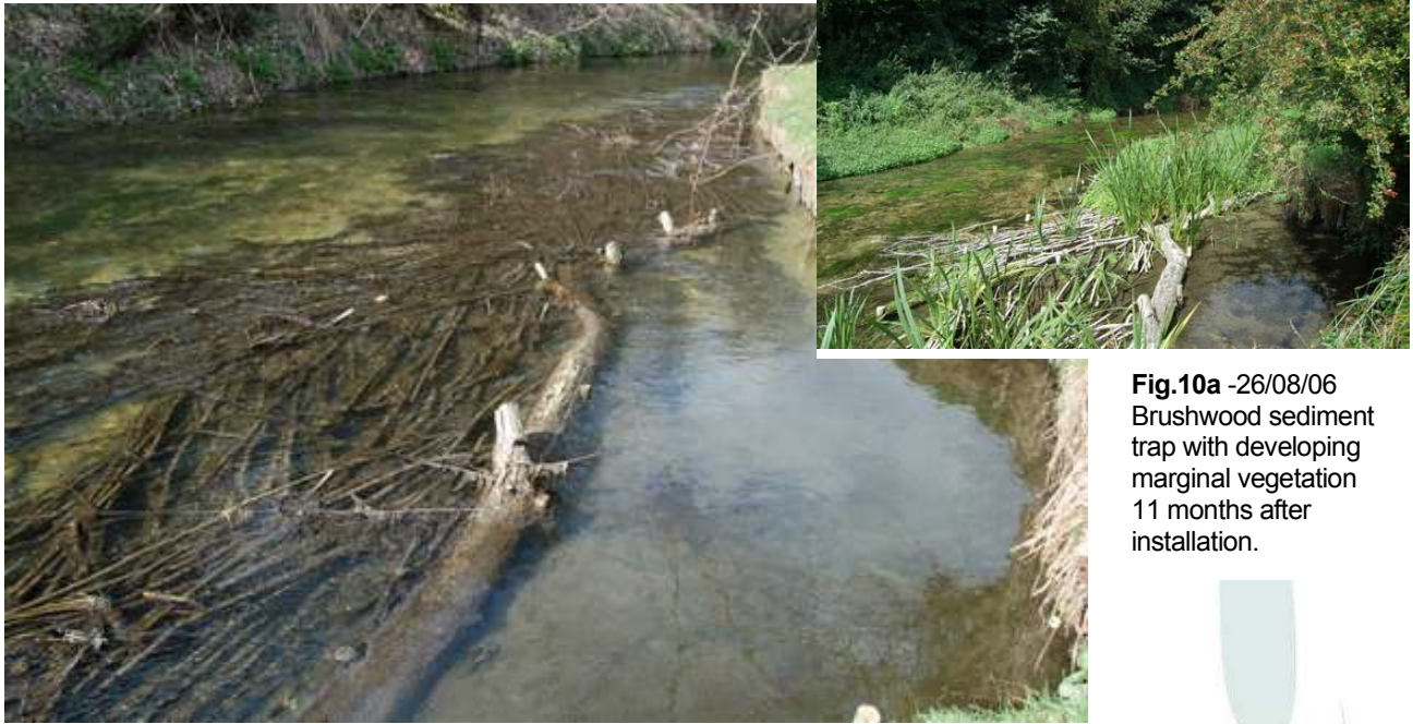
Fig.10 26-03-06 Spring 2006 Brushwood marginal mattress with light organic sediment accretions 6 months after installation. The anticipated heavy inorganic accretions failed to materialise due to a drought winter and almost total lack of floods.
