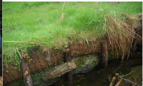
Fig 15a – Composite LWD/Coirnet Bank revetment.
