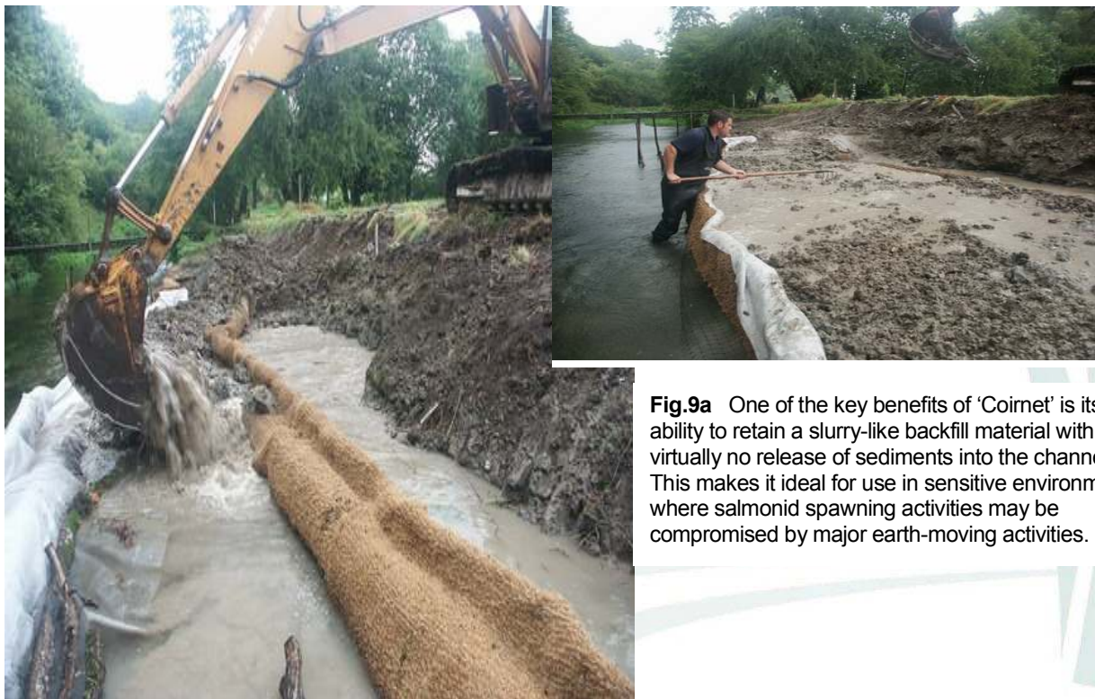
Fig.9 CBE's 'Coirnet' bank revetments being in-filled to form a new low-level riparian flood berm. The borrow pit being excavated to the rear will be retained as an off-line pond.
