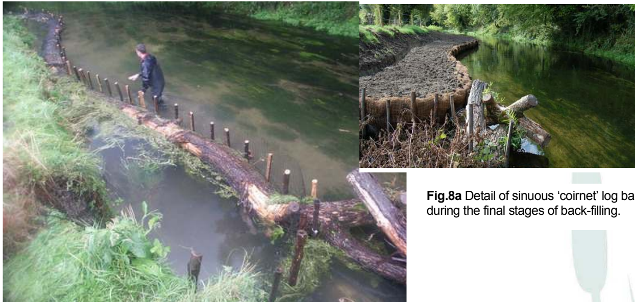
Fig.8 Sinuosity can be achieved by the careful selection of on-site woody material.
