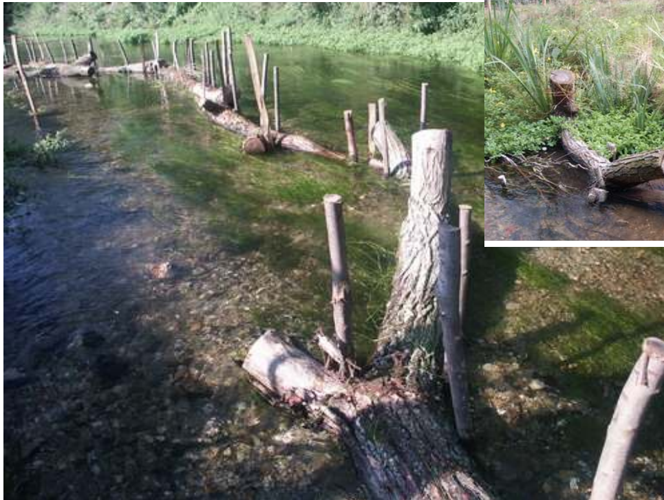
Fig.7 Mark out the line of the new bank face ‘toe’ using carefully selected woody material, where available. This can be live or dead depending on need and is not species critical.
